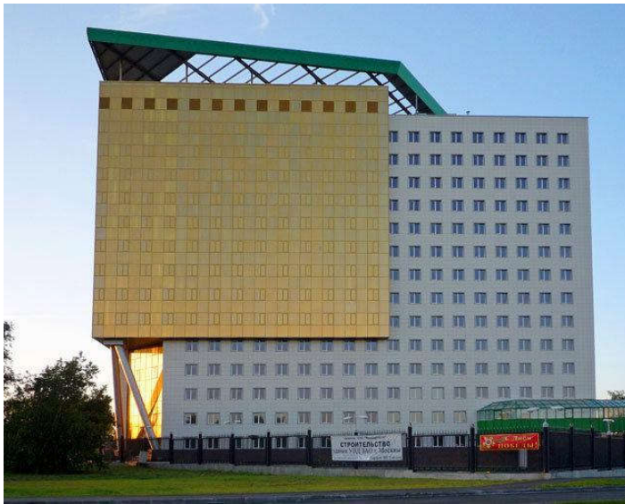
Figure 1.1 Police building of western administrative district of Moscow equipped with R65-BP system.
